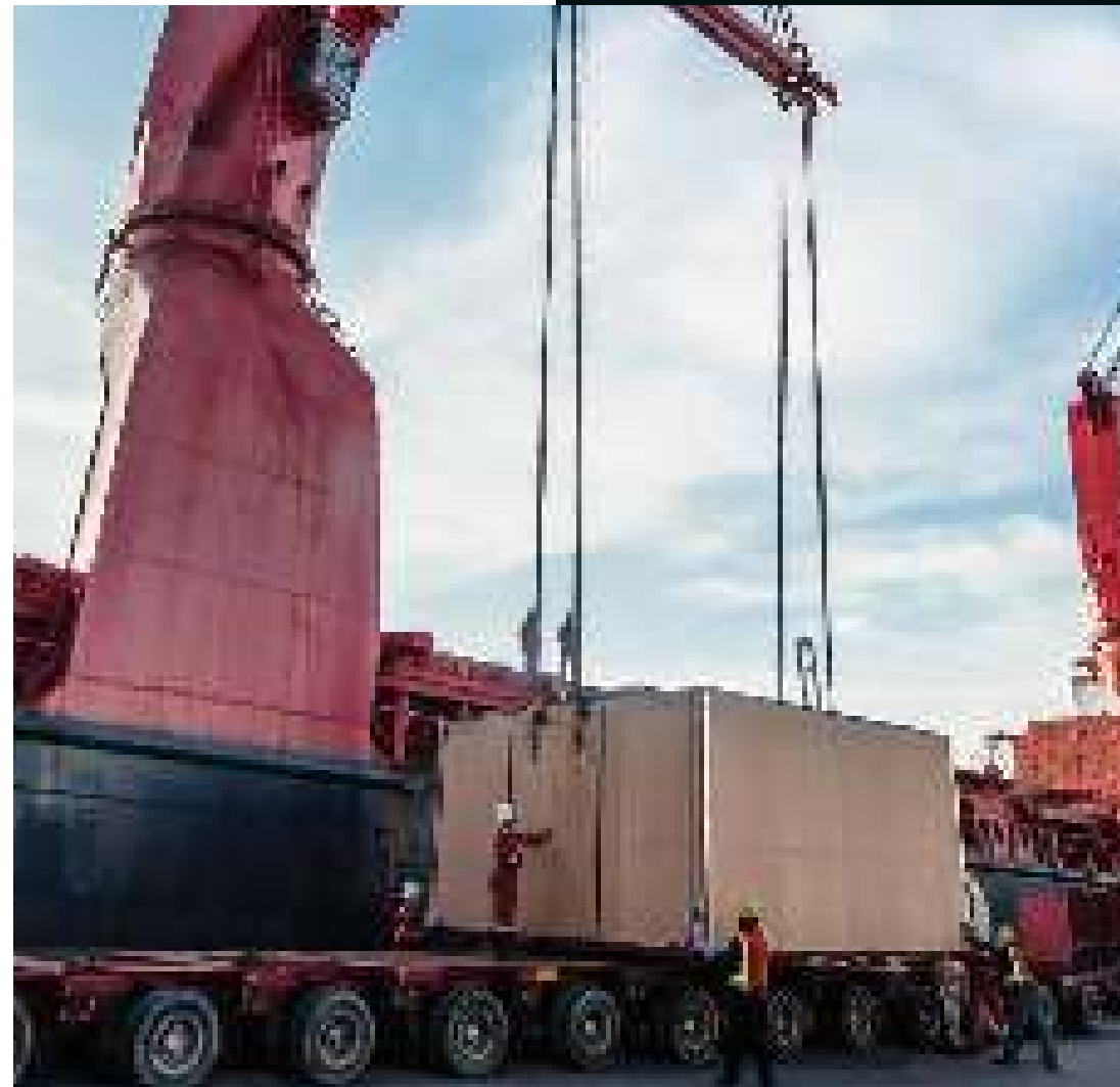
Heavy Lift Supervision Inspection Services
